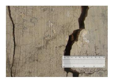
With "severe" wall cracks (15 to 25 mm wide) window and door frames may be distorted, floors slope noticeably, walls lean or bulge, some loss of bearing in beams, service pipes are probably disrupted and a gap of up to 20 mm between ceiling cornices and walls may appear.
